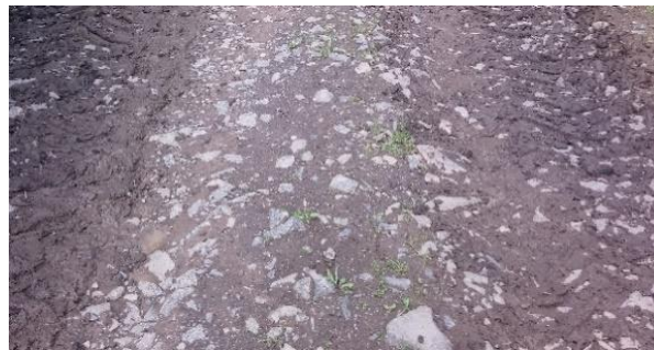
Fig. 1. General view of the forest road condition
