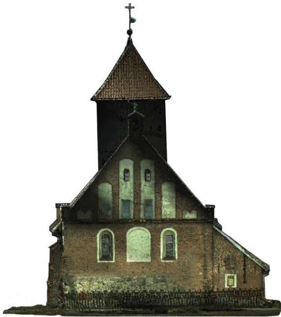
Fig. 1. Eastern facade of a rural church in the form of a point cloud with superimposed photographs
