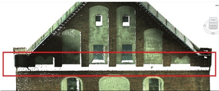
Fig. 3. Cornice - shadows in the point cloud on its upper surface
