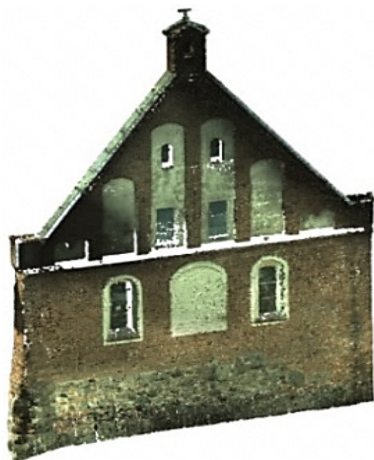
Fig. 2. Eastern wall in the form of a point cloud, including photographs
