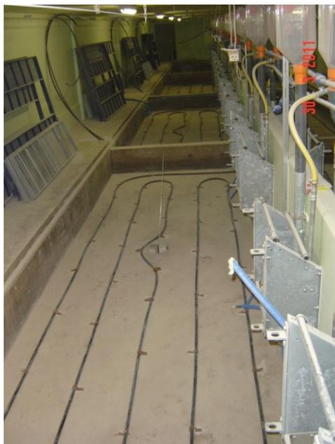
Fig. 1. Heat pump collector in under floor manure canal
