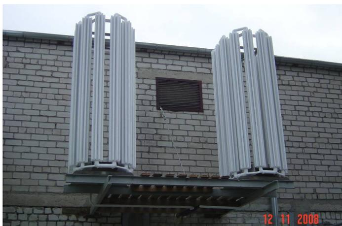
Fig. 2. Evaporators of heat pump IS 81
