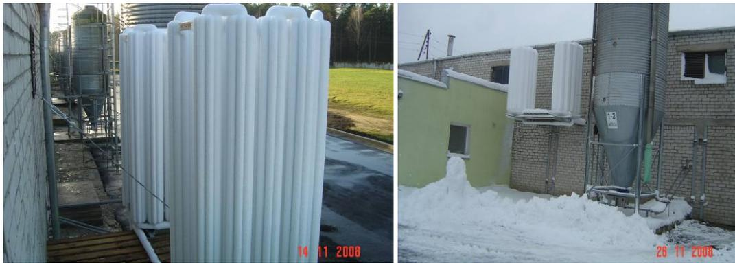
Fig. 6. Evaporators covered with hoarfrost during exploitation
