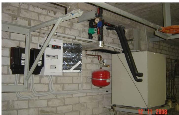
Fig. 3. Compressor of heat pump IS 81 with heat exchanger (container on the right), control unit and measuring equipment (on the left)
